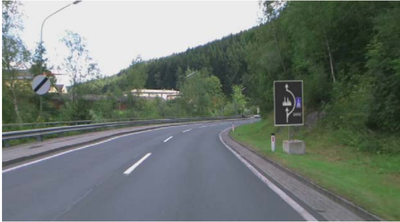
Fig. 12. Traffic scene with the design UOT on the right and a speed limit end sign on the left
